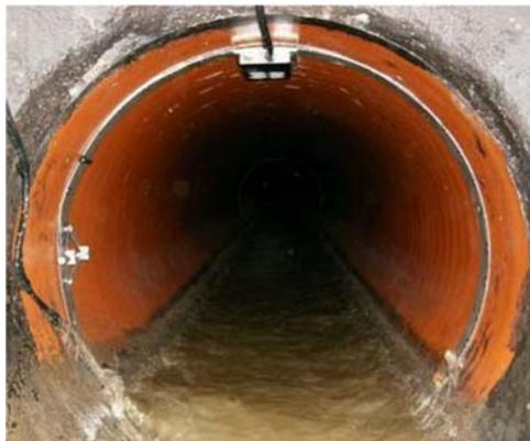
Figure 5.2: Flow measurement using the velocity-area method
